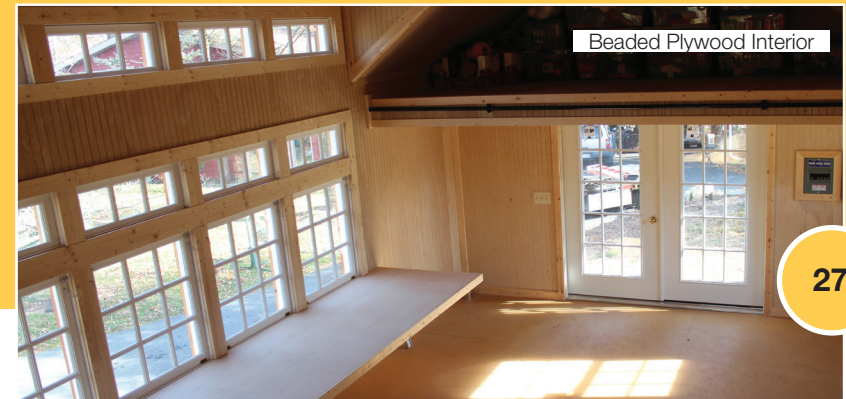
Tongue & Groove Pine Interior and Floor
