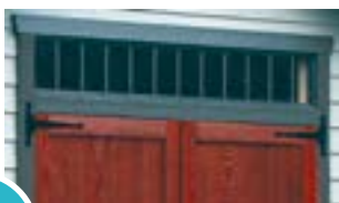
Transom Window Above Door
